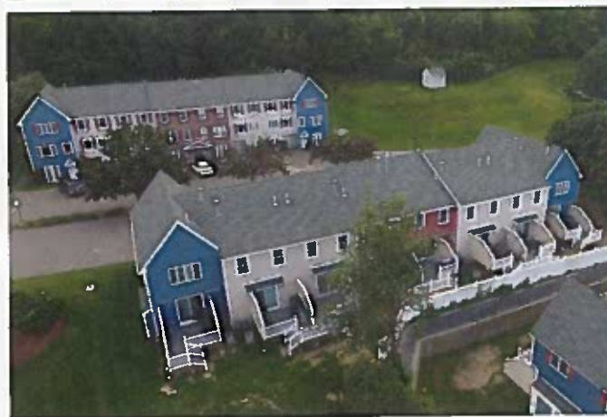
Top Photo: Overlooking Fox Meadow Condominiums in Leominster, Mass., you can see the completed envelope project by Adam Quenneville Roofing & Siding of South Hadley, Mass. Bottom Photo: Adam Quenneville Roofing & Siding finished the entire envelope project two months ahead of schedule. The project involved 17 buildings at Fox Meadow Condominiums in Leominster, Mass.
